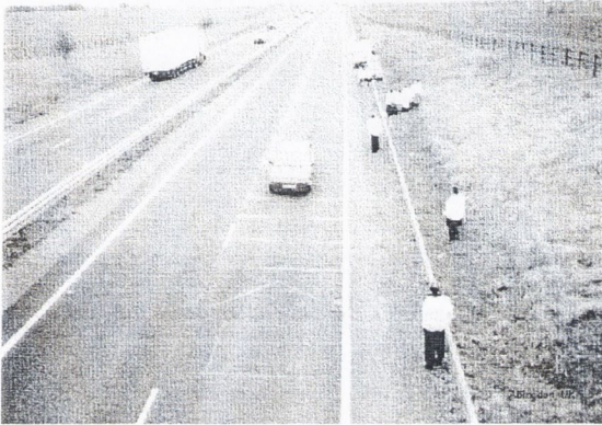
(a) Capacitive strip multi-sensor array at Abingdon, UK
