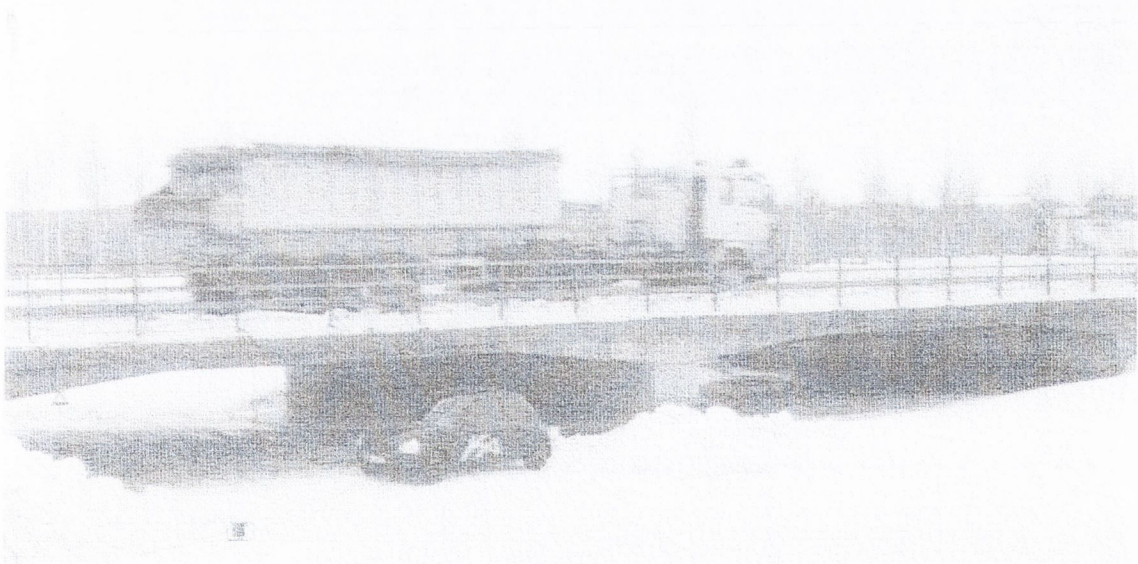
Figure 8.19 - Side View of Luleå Bridge
