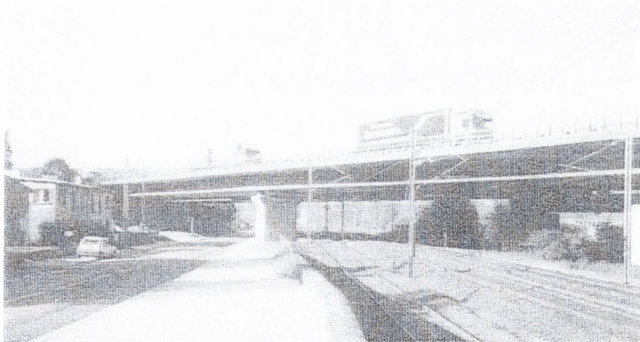
Figure 8.30 – Side View of Belleville Bridge
