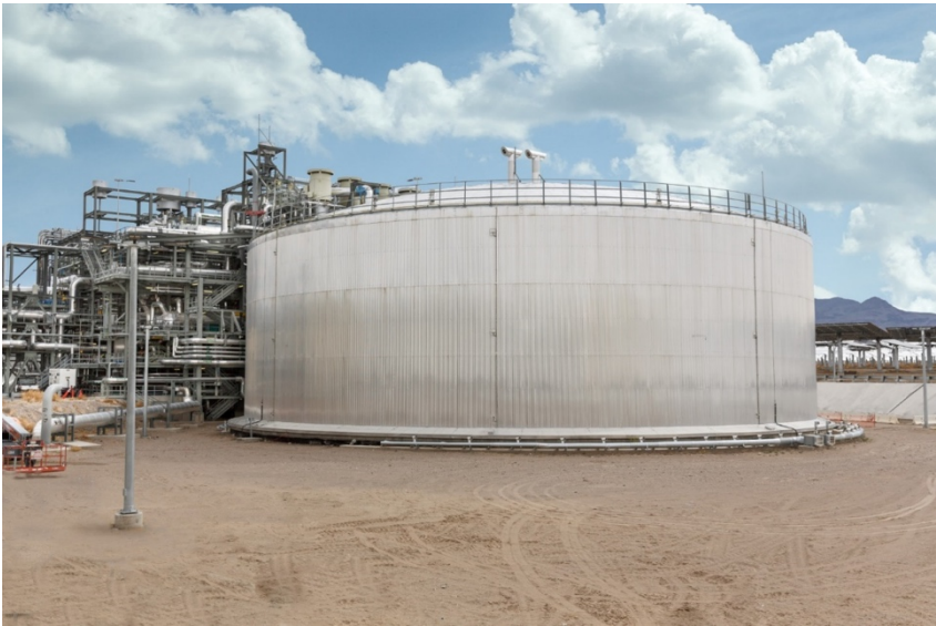
Figure 2.8 Salt tank for heat storage in CSP (Source: U.S. Department of Energy).
