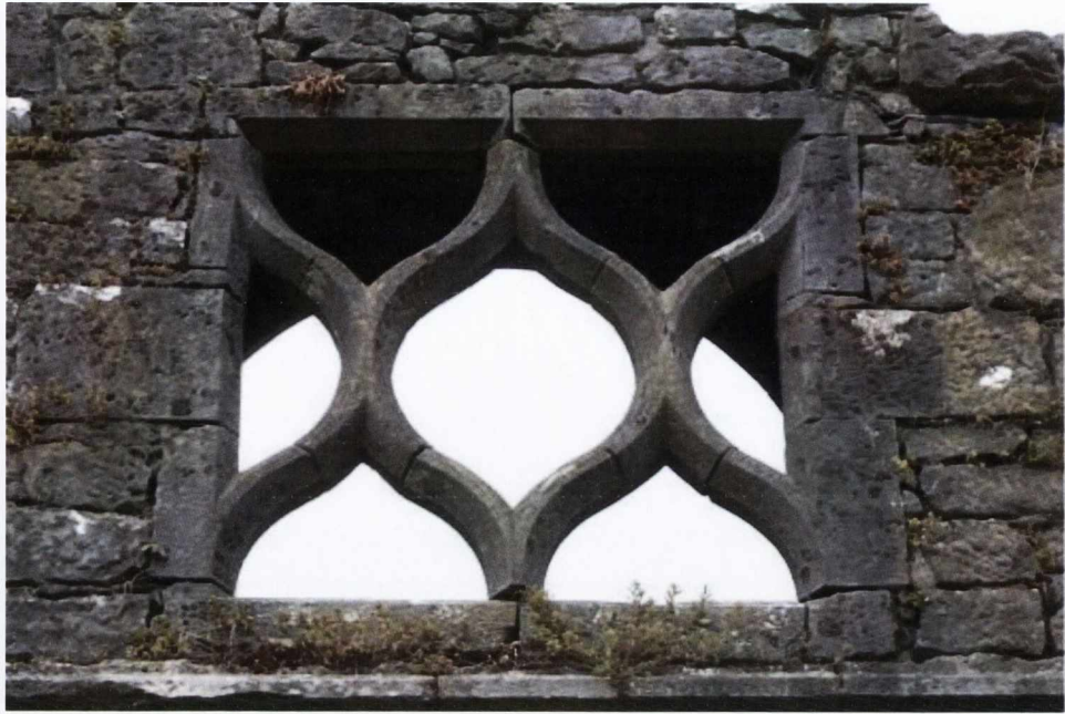
Figure 4.11 Nave south wall, Augustinian friary, Callan
