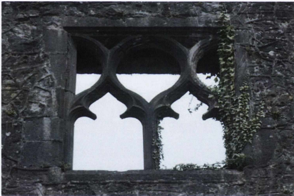
Figure 4.12 Nave north wall, Carmelite friary, Loughrea
