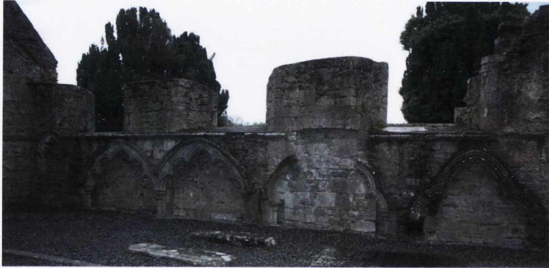
Figure 4.41 Tomb niches and piscina, south aisle south wall, St. Mary's collegiate church, Gowran
