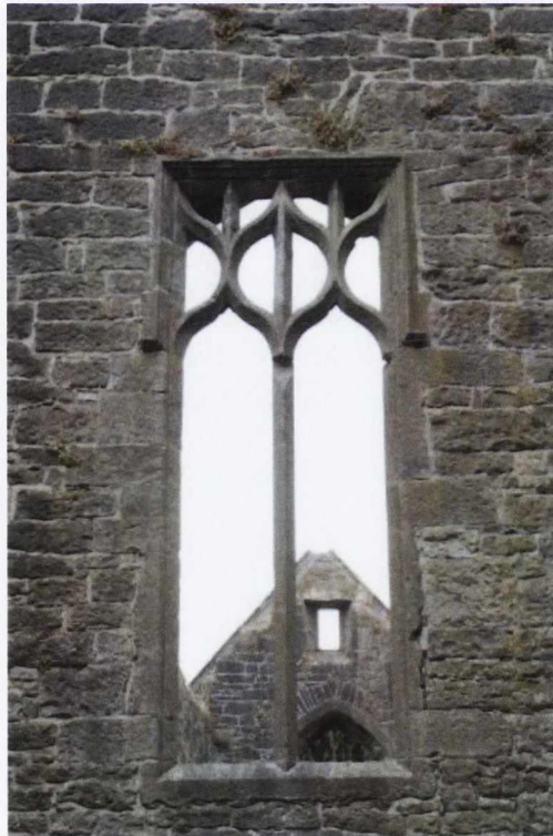
Figure 4.7 North aisle west window, St. Mary's parish church, Callan
