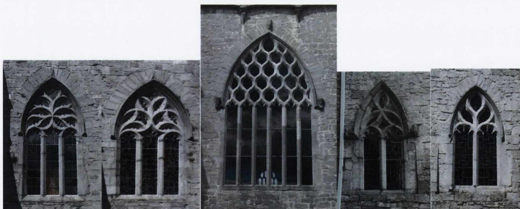
Figure 4.22 East windows of the chancel and transepts, Holycross Cistercian abbey (relative scaling approximate)
