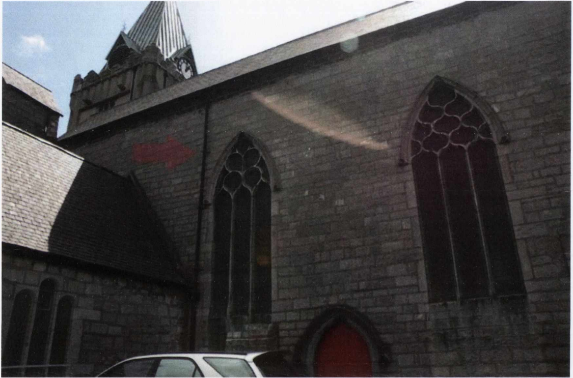
Figure 5.12 St. Nicholas collegiate church, Galway: north aisle of the nave. The arrow marks the approximate position of Leask’s ‘very slight obliquity’
