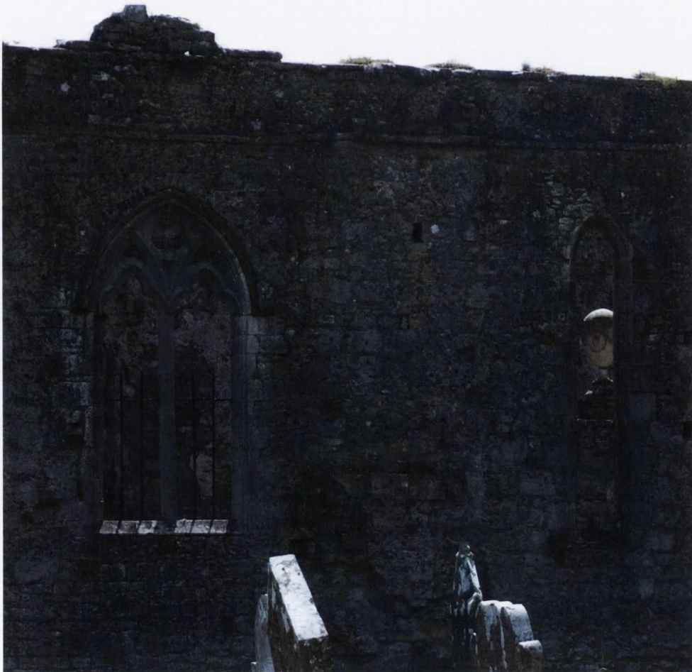
Figure 5.19 Athenry Dominican priory: chancel north wall details
