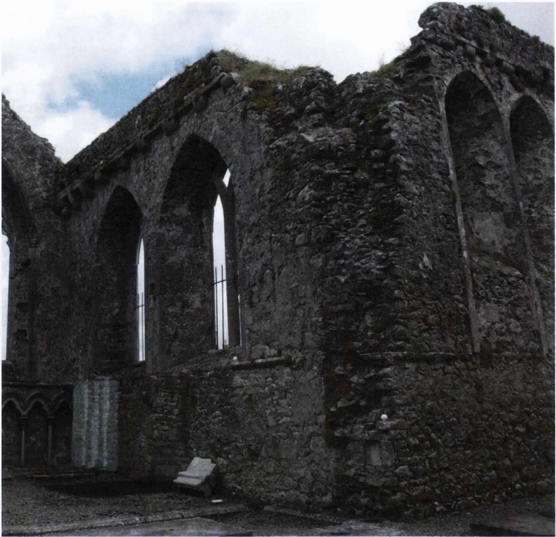
Figure 5.52 Athenry Dominican priory: north transept east wall, internal view. The cyan highlight indicates the approximate location of the blocked doorway. Note that the masonry on the transept east wall below the stringcourse matches and joins seamlessly with the masonry inserted at the junction of the transept east wall and the chancel north wall for the construction of the crossing tower in the fifteenth century.
