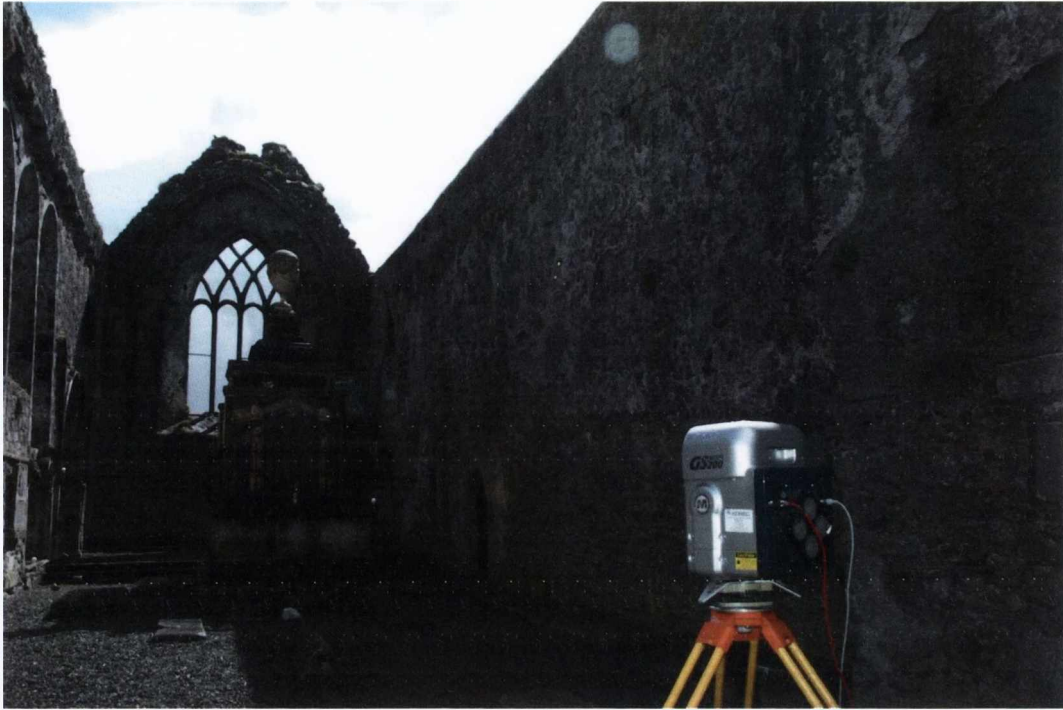
Figure 5.18 Athenry Dominican priory: internal view of the chancel from the crossing. Note the different lean of the wall above the arches surrounding the lancets and the presbytery windows.
