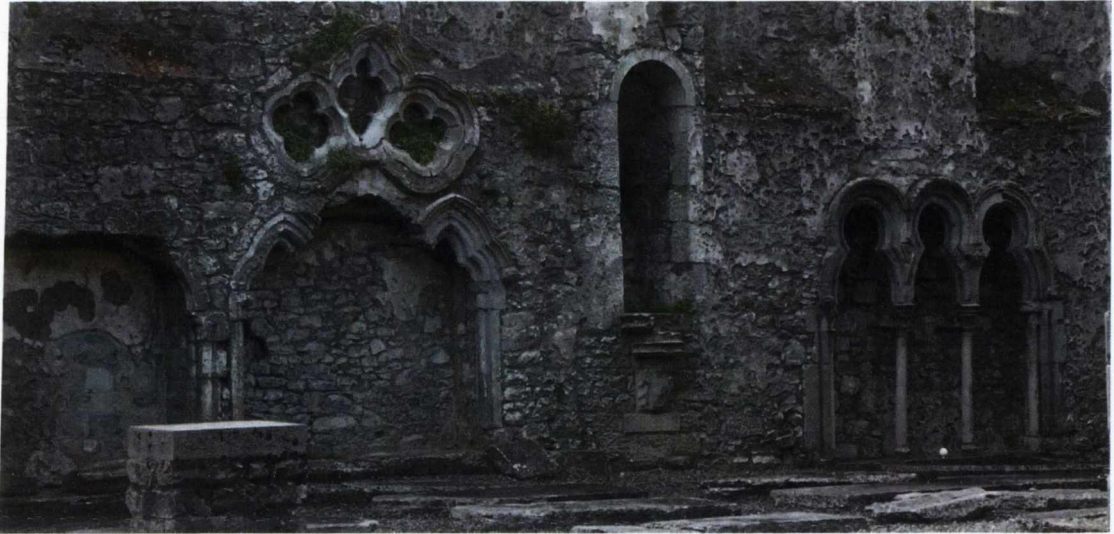
Figure 5.39 Athenry Dominican priory: nave south wall
