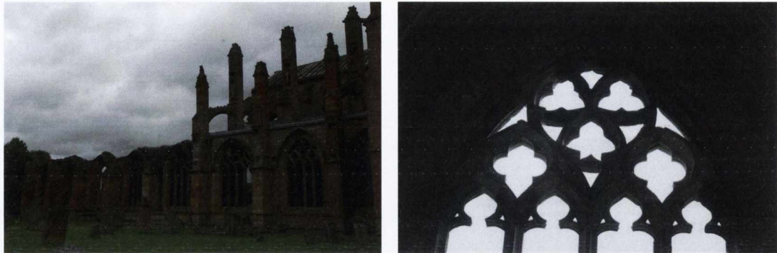
Figure 7.19 South aisle from the south east (left) and tracery including triangle with curved sides, seventh chapel from the west, south aisle (right), Melrose Cistercian abbey
