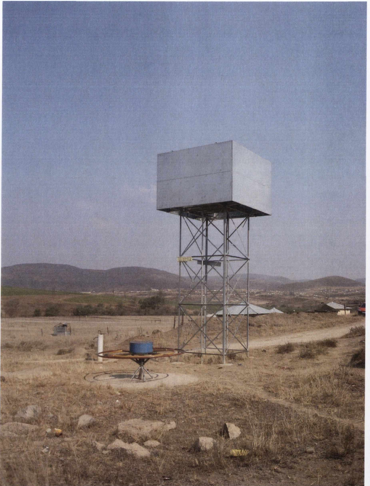
Fig 7.1: A PlayPump without advertisements, and with no water in the tank, visited by the author in KwaZulu Natal in August 2010. See fig 7.5 in this chapter for photographs of all 10 installations visited in the region.
