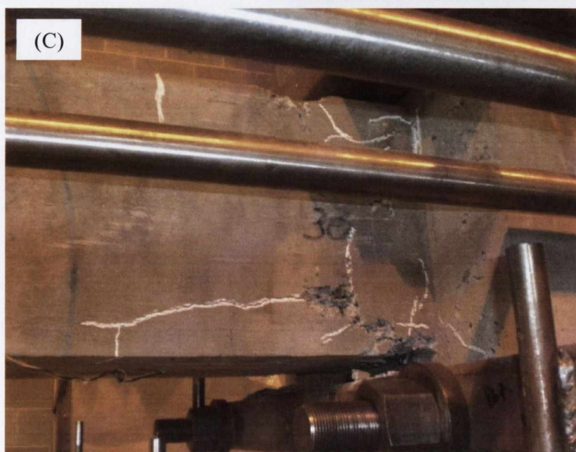
Figure 4.11: Photos: (A) – (C) Specimen JD1: Damage Post 30mm Displacement Cycle
