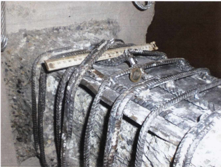
Figure 4.12: Visual Post Test Specimen Damage
