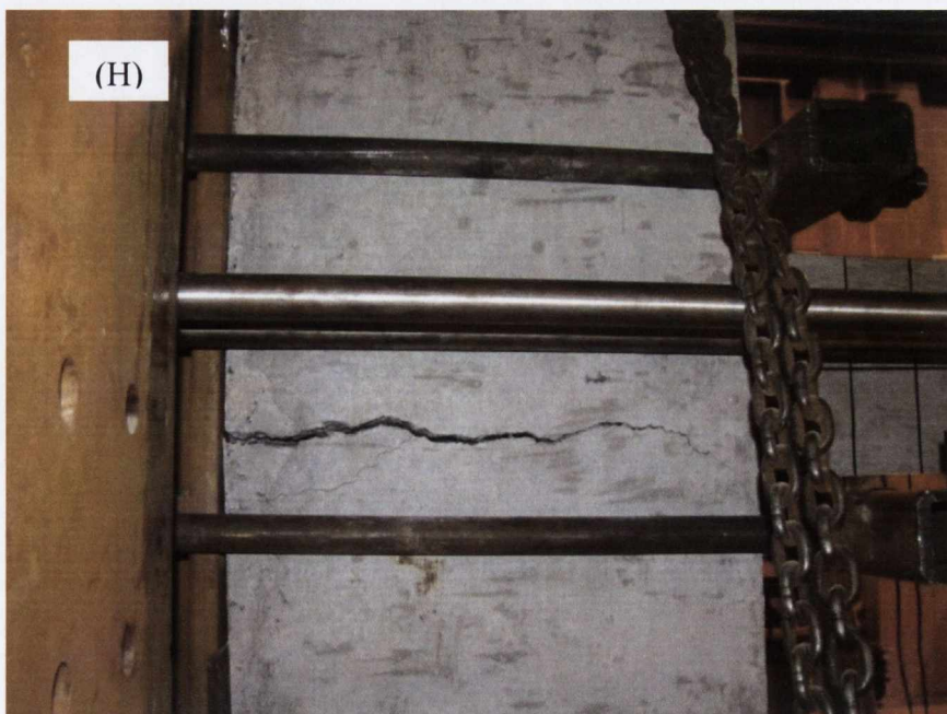
Figure 4.11: Photos: (G) & (H) Specimen JD5: Base Cracks, Face 4 & Face 2
