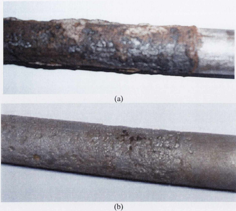
Figure 5.21. Corroded reinforcing bar before and after cleaning
