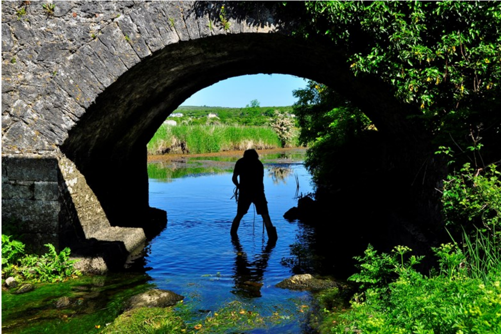
Figure A.4: Discharge measurement taken in the Fergus River at Crossard Bridge.
