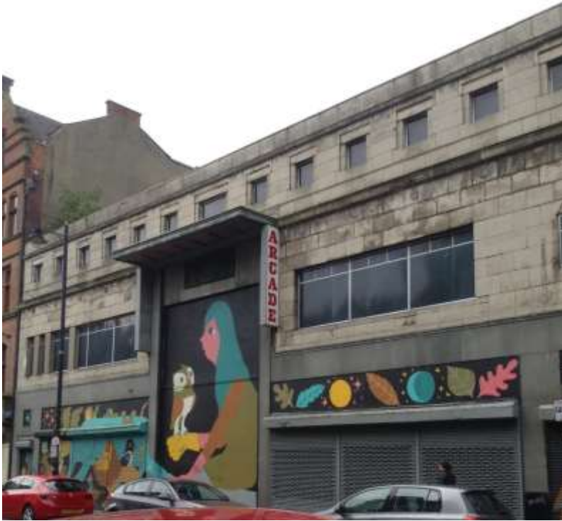
Figure 28: Located at North Street Arcade (Photograph by the researcher, May 2016)
