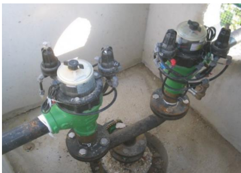
Figure 2-6. Pumping station (head control unit)
