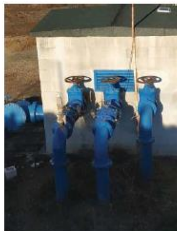
Left: The REDAWN pilot plant constructed in the irrigation sector, which worked for the 2019 irrigation season
