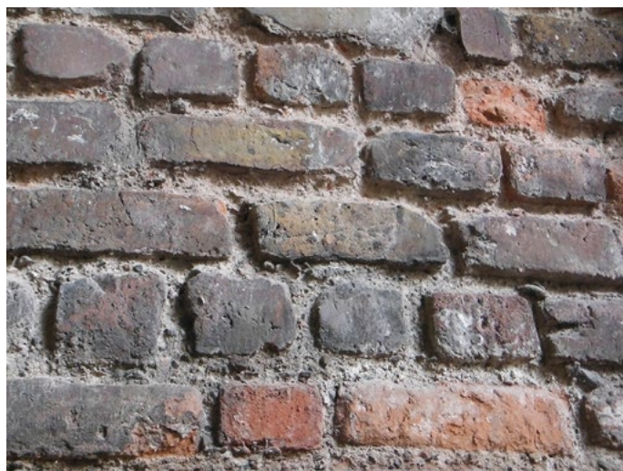
Figure 5 Detail of the brick bond in the back wall. Photograph by Sara Pavia.
