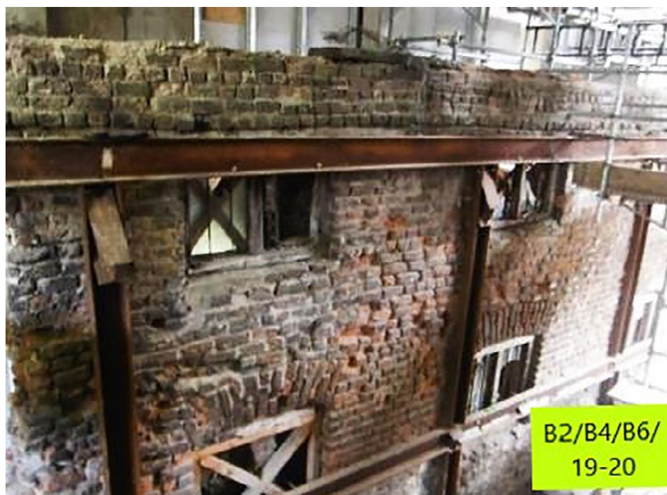
Figure 2 Samples taken from the back wall, probably built before 1634. Photograph by Sara Pavia.
