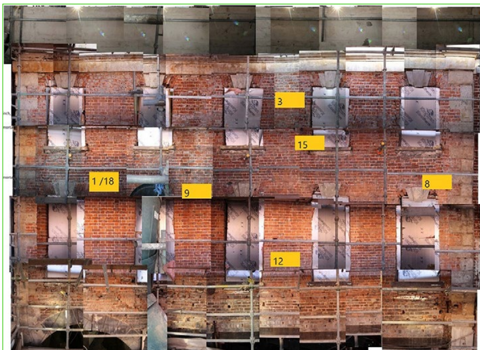
Figure 1 Fade Mansion during restoration work in 2018, showing the original brick fabric and the sampling. Published with the permission of Neil Crimmins of Cathal Crimmins Architects.
