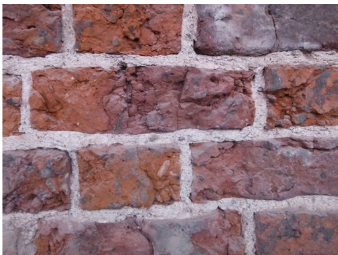
Figure 4 Detail of the brick bond in the façade walls. Photograph by Sara Pavia.
