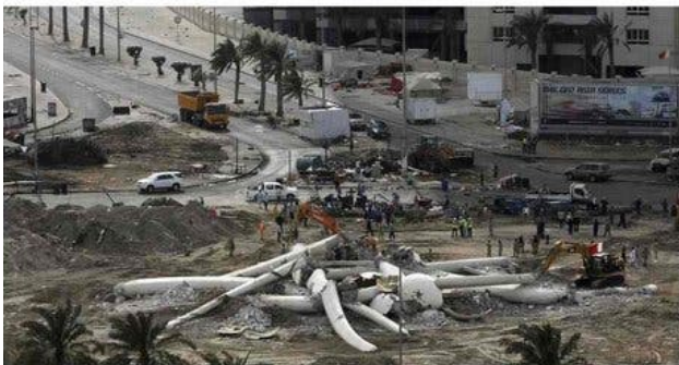
Image 46: Image sequence of demolition Hamad I Mohammed/Reuters. [online image].
