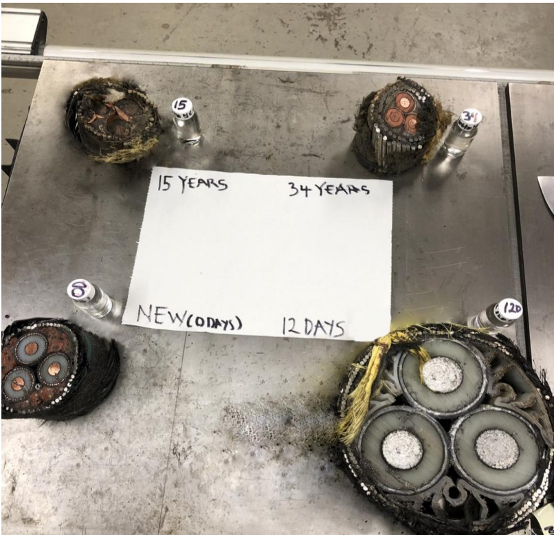
Figure 15a: A picture of the 4 subsea power cables
